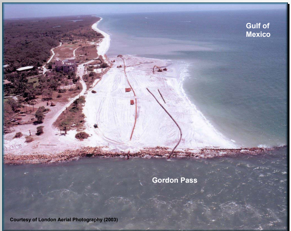
PROJECT UNDER-CONSTRUCTION MAY 2003
